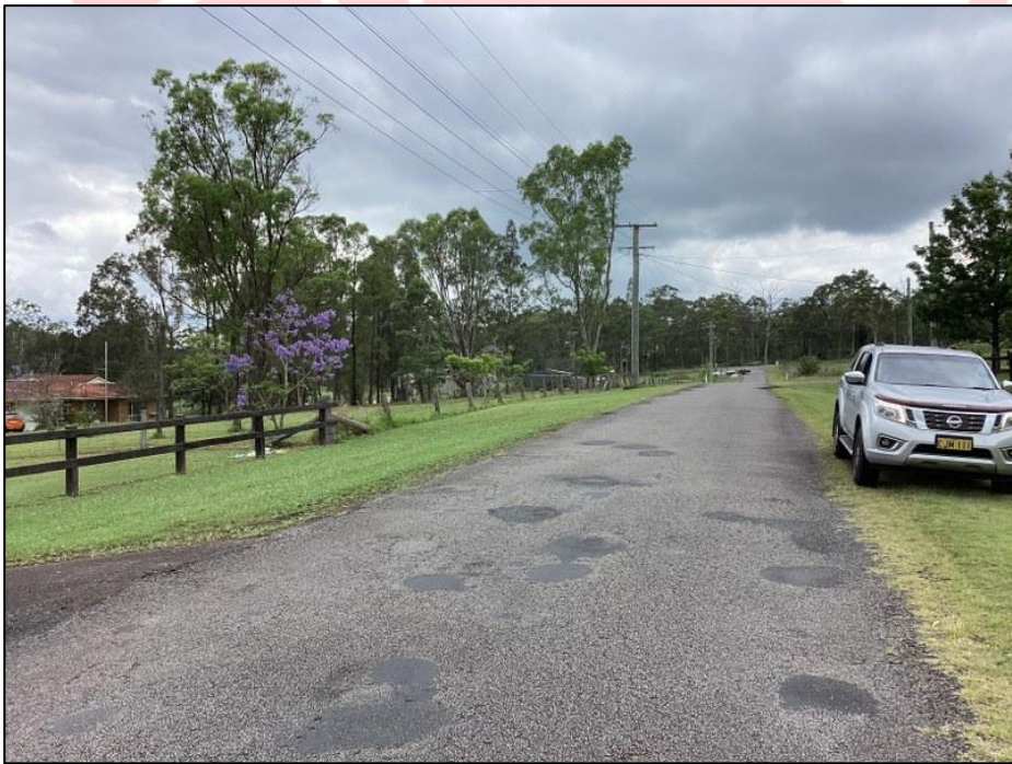
Plate 2 (P2) Access along Horns View Street
