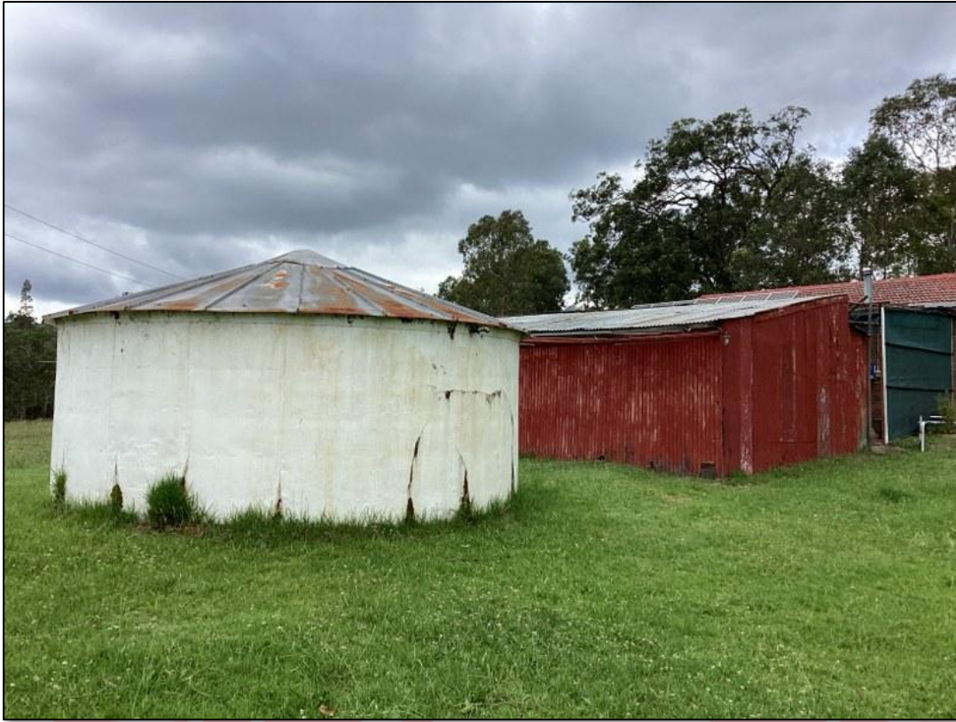
Plate 7 (P7) Existing static water Supply for existing dwelling
