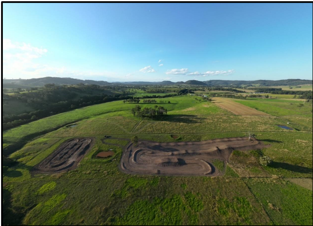
Flyover Photo – Constructed Motocross Tracks at No 47 Horton Cl Glen Martin (Apr 2024)
